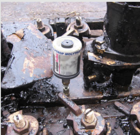
Lubrication of gear rack
